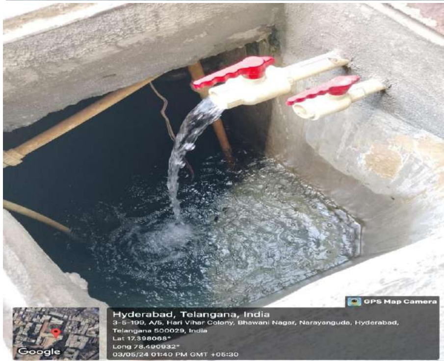
Construction of Sumps for storage of water near U.G Block
